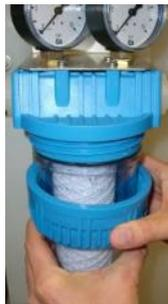
4. Unscrew the blue union nut. Pull it away (downwards) together with the filter casing.
